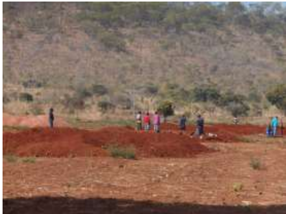
Men at work; digging of the foundation
